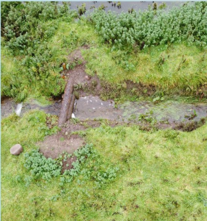
Figure 14: Leaky dam structures along with high flow diversion channel and flow attenuation pond after a large flood event. Left: single leaky dam measure, right: two leaky dams with channel and pond.
