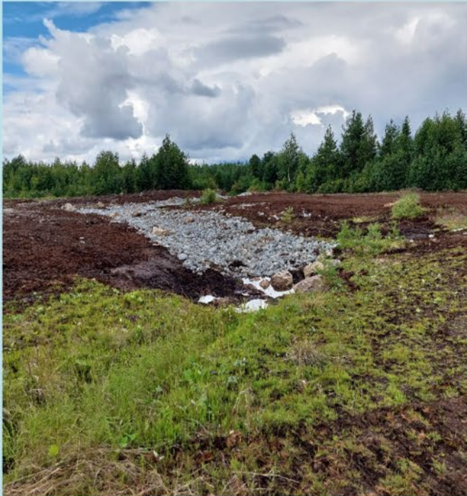
Figure 8: Completed construction of a ditch conducting water towards the built wetlands and peat restoration area.
