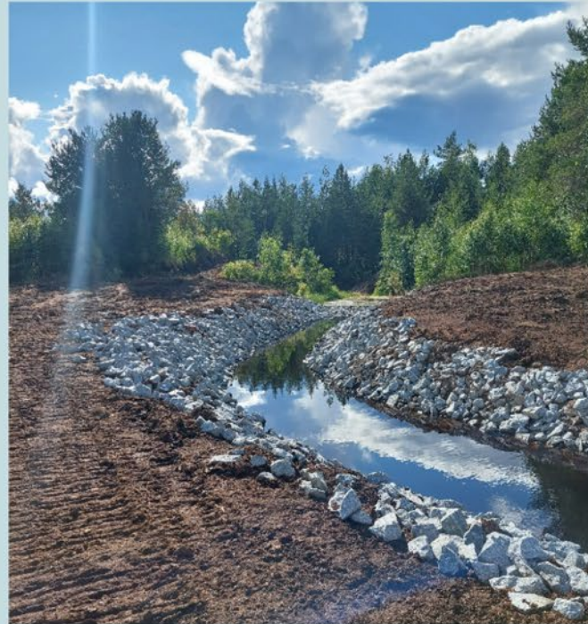
Figure 8: Completed construction of a ditch conducting water towards the built wetlands and peat restoration area.
